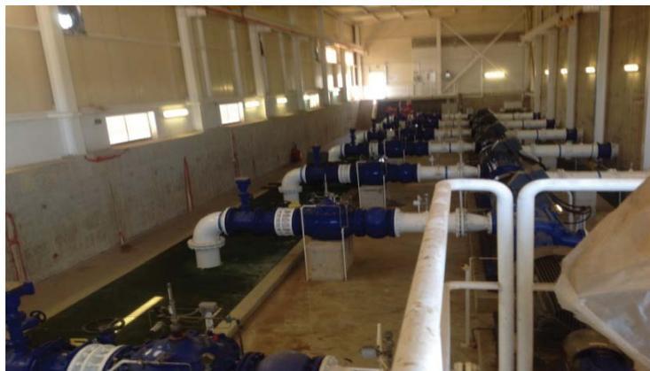
Fig. 5 Treated water pumping station. Source: (Personal photography, June 2017).
