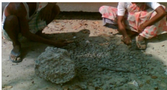
Fig. 1 Crushing of concrete waste into aggregates.
