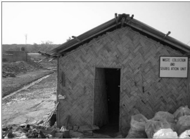
Fig. 4 Waste collection and segregation unit within a drill site in Assam north east India
