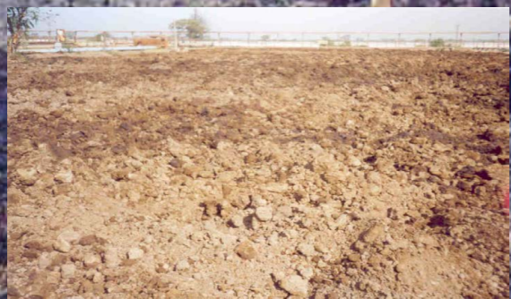
Fig. 11 Site after process completion
