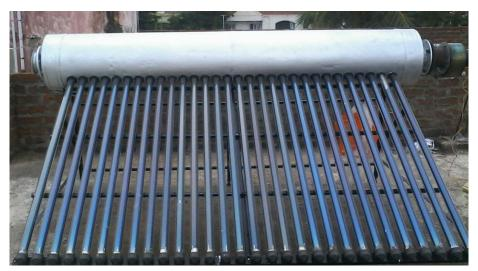
Fig. 1 The evacuated tube absorbs solar energy.
