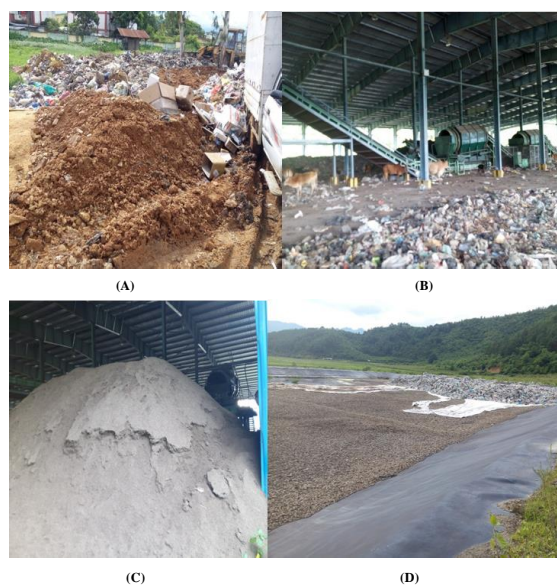
Fig. 1 (A) Earth cover at Porompat landfill; (B) Compost plant at Lamdeng landfill; (C) Compost at Lamdeng landfill; (D) Layer sheet below solid waste at Lamdeng landfill.
