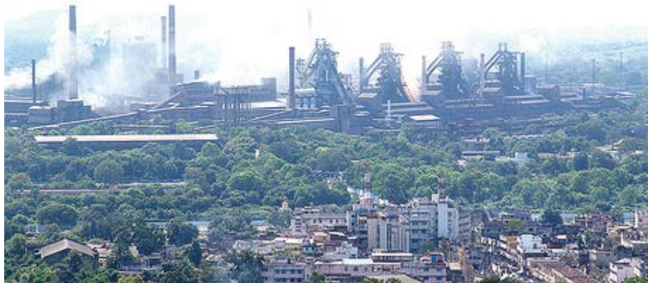
Fig. 4 Overview of Rourkela steel plant.
