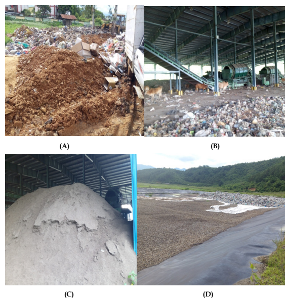
Fig. 1 (A) Earth cover at Porompat landfill; (B) Compost plant at Lamdeng landfill; (C) Compost at Lamdeng landfill; (D) Layer sheet below solid waste at Lamdeng landfill.
